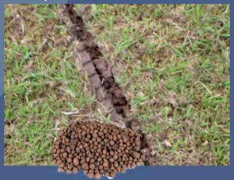
View of cut channels with infill of Lytag
